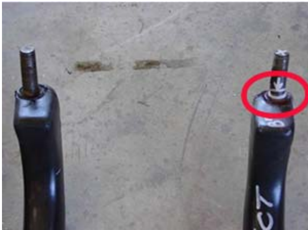
Location of cracking
